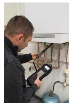
Ambient CO checking
