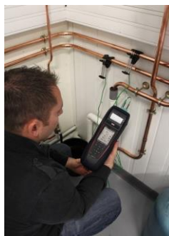
DHW network temperature
