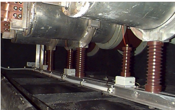
Fig. 1: Permanent coupler installation
